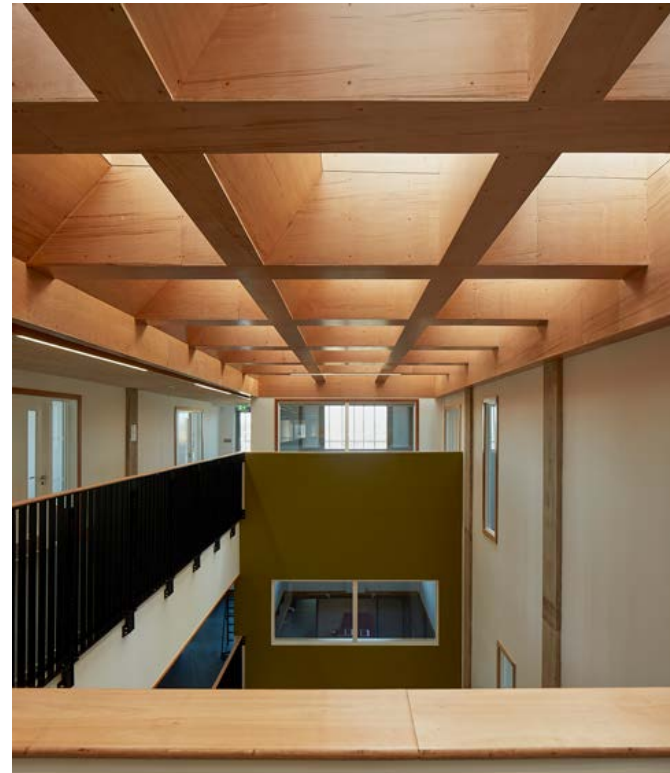
Timber elements combined with the LAMILUX Glass Skylight FE Passivhaus emphasise the sustainability of the Eco Business Centre in Bicester, England.
