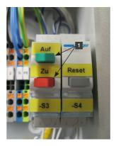
Move the roof access hatch to the desired position by means of the emergency control button (1) while keeping visual contact or secured by safety personnel. The emergency control buttons (1) are marked accordingly with "OPEN" and "CLOSED".
