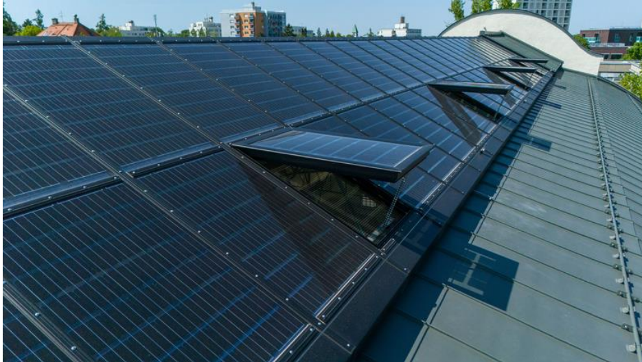
Daylight, fire protection and energy generation combined through Glass Roof PR60
