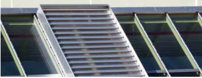
NSHEV type SMOKEJET in a shed roof
