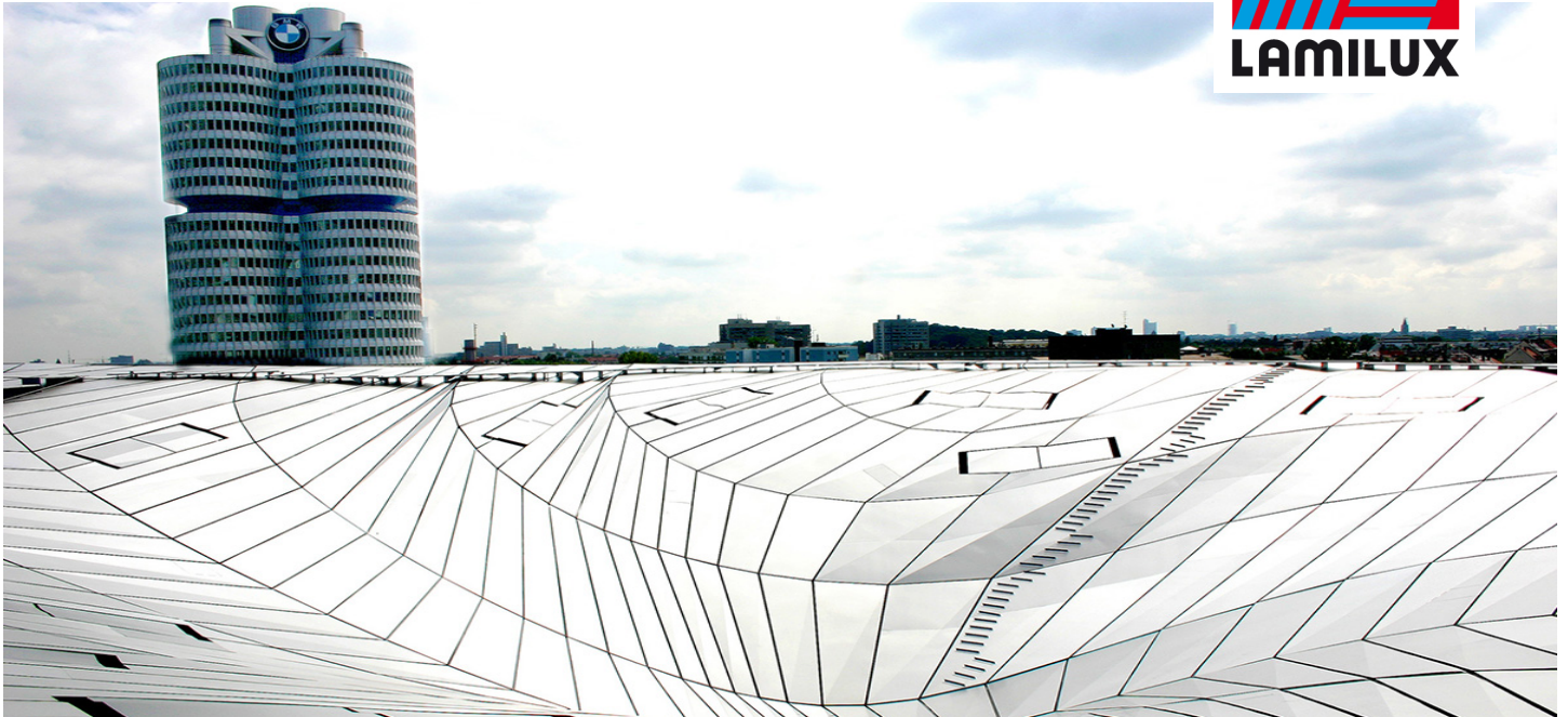
BMW Four Cylinder Building, Munich
