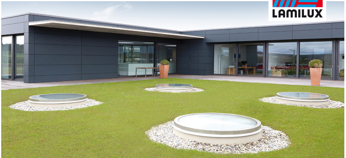
Administration and Logistics building, Ötisheim
