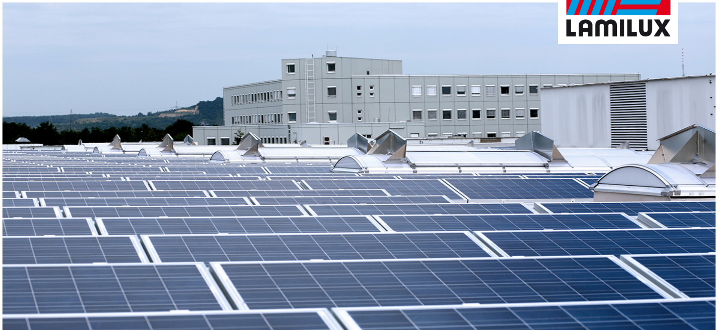
Schneider Electric, Regensburg, Germany
